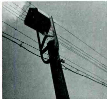
Fig. 3. View of frame atop one pole shows metal shield to keep ice off insulator.
